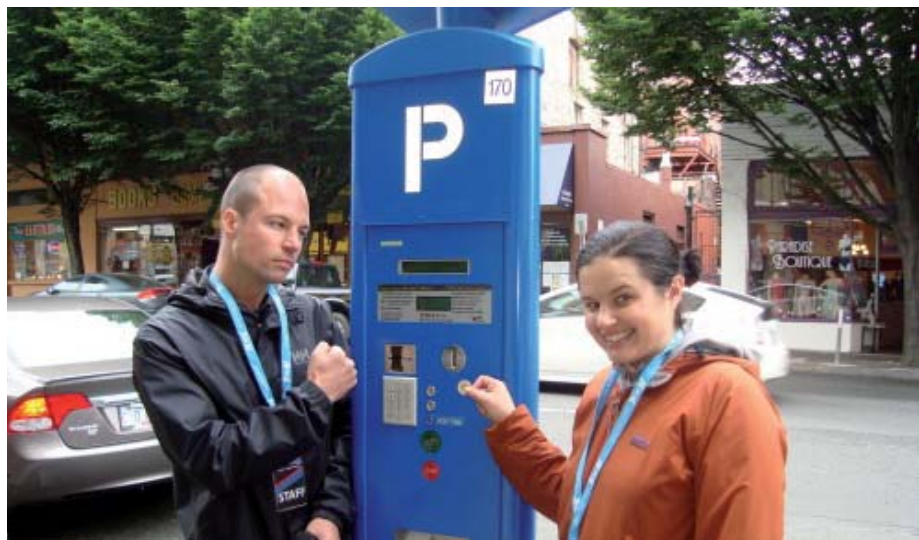
Example of kiosk-style meter used in downtown Victoria. (Source: www.koolmornings.wordpress.com )
