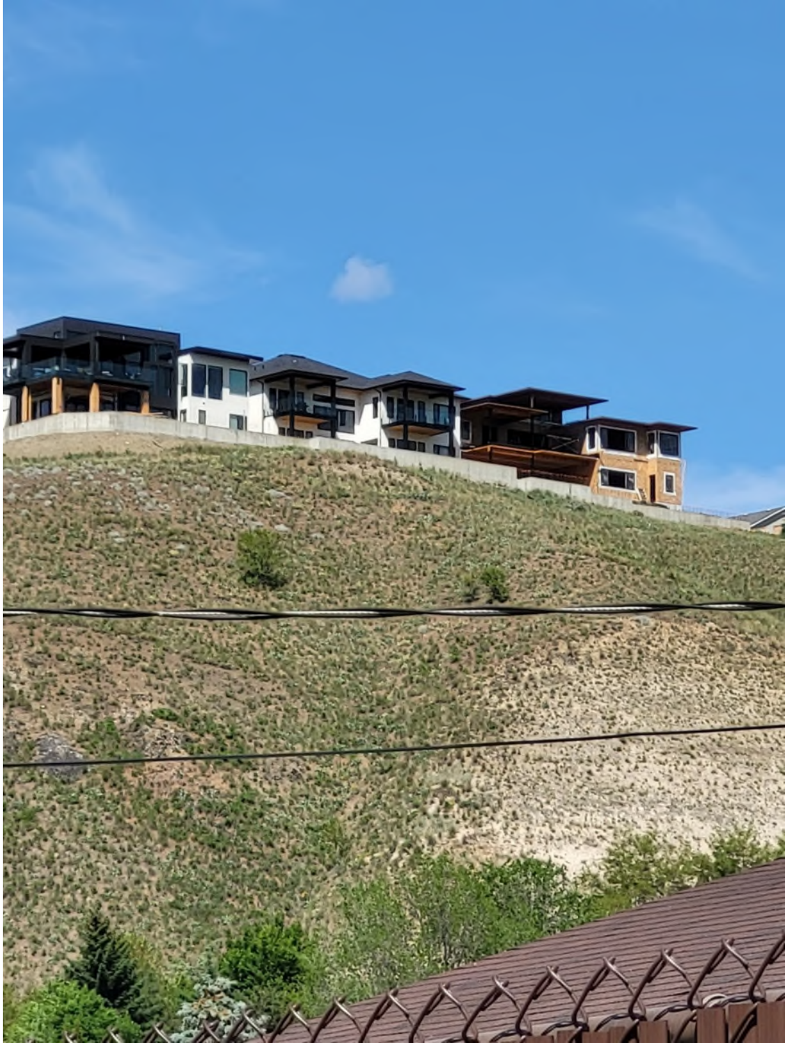
Subject property is the centre white single family dwelling (900 Mt. Griffin Road)
