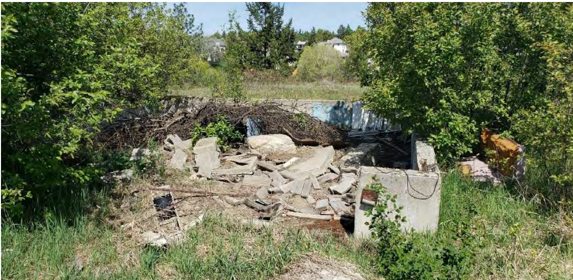
Photo 4 Building foundation and debris (to be removed) along west boundary of the Site. Aspect north.
