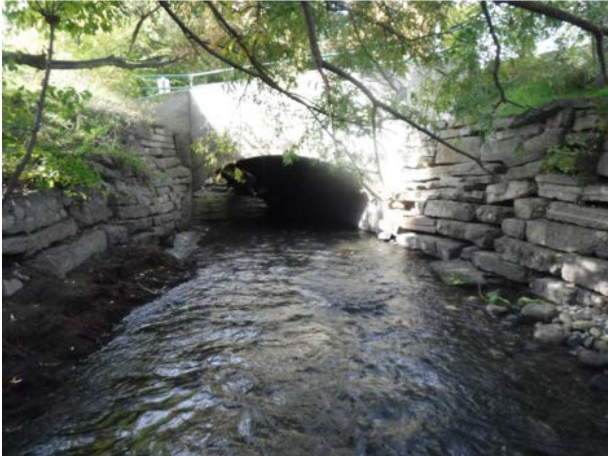
Figure 8.11 Lower Vernon Creek at 43 rd Street culvert crossing, facing downstream.
