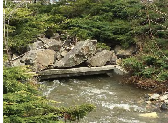
2018 – Inlet box culvert 48 th Avenue crossing
