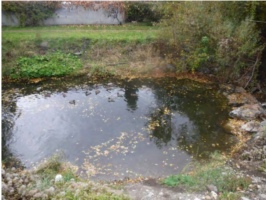
Photo 8.1 Sediment trap downstream of Pleasant Valley Road crossing (NHC, 2019).
