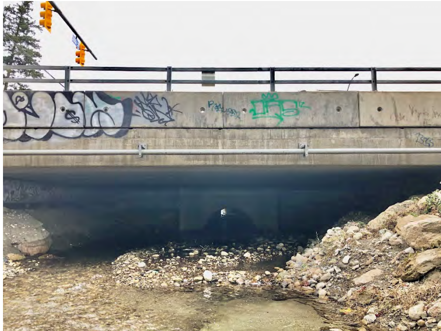
Photo 8.3 Sediment deposited at outlet of 48 th Avenue crossing (NHC, 2019).
