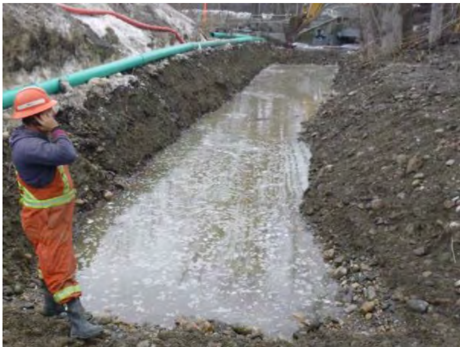
Photo 8.2 Sediment removal between 48 th Avenue and 20 th Street crossings (CoV, 2018).
