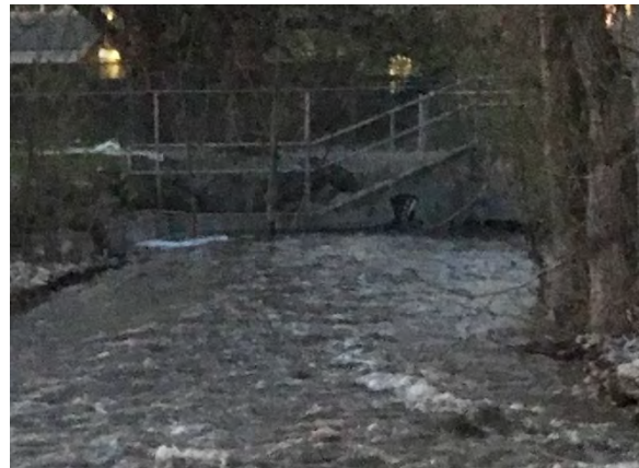
2018 – Inlet box culvert second 20 th Street crossing
