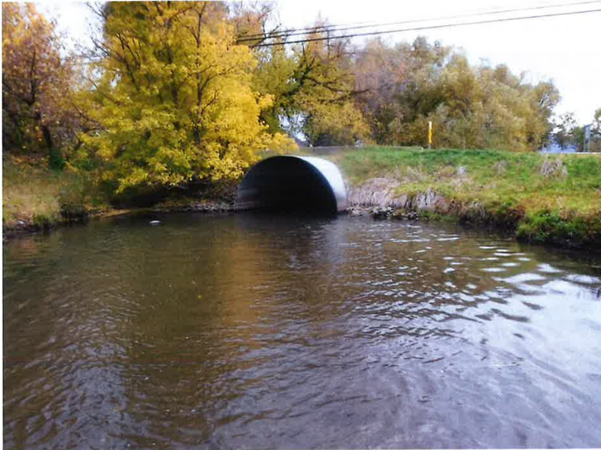
Figure 8.15 Lower Vernon Creek at Lakeshore Road culvert crossing, facing downstream.
