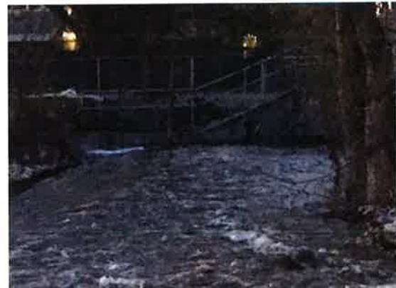
2018 – Inlet box culvert second 20 th Street crossing
