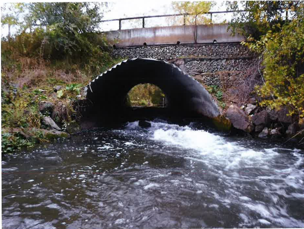
Figure 8.13 Lower Vernon Creek at Okanagan Landing Road culvert crossing, facing upstream.
