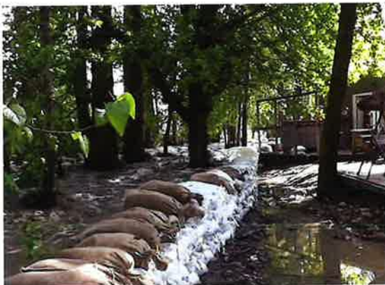
2018 – Sand bag wall behind 4905 20 th Street
