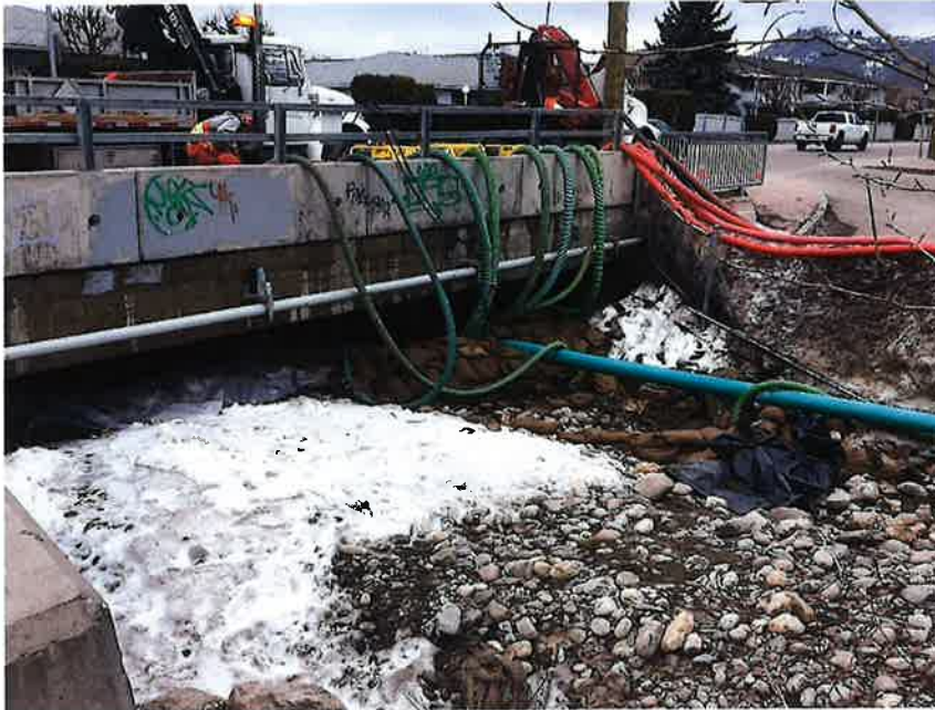
Figure 2.2. Sediment deposited at the outlet of 48 th Ave Crossing prior to dredging (CoV, 2018)
