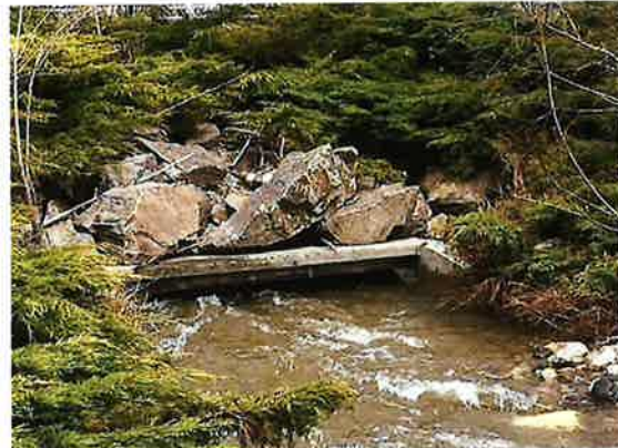
2018 – Inlet box culvert 48 th Avenue crossing
