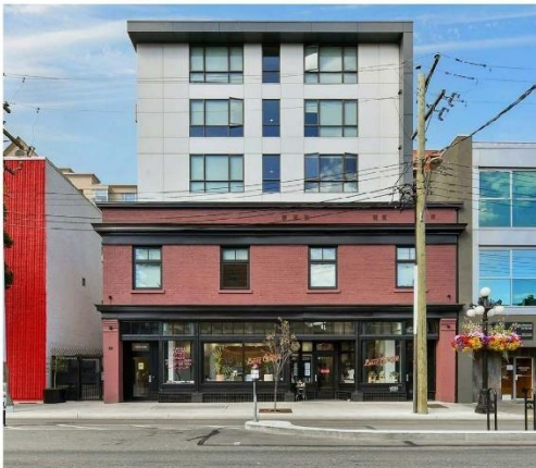
Figure 14: Encourage retention and revitalization of heritage buildings.
