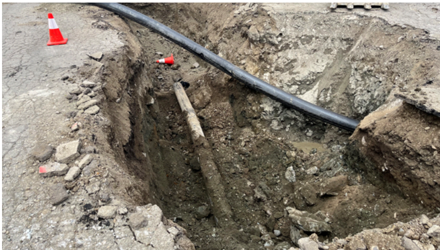
Sewage line work in progress
