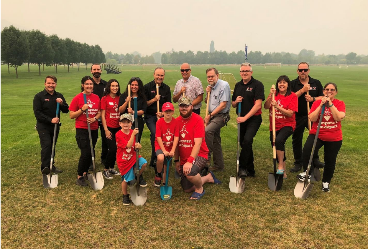
Above: The ground is broken at Marshall Field Park for Vernon’s new Canadian Tire Jumpstart Charities’ Inclusive Playground, to be opened in Fall 2021.
