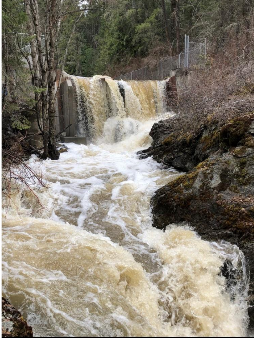
Upper BX Creek sediment basin – May 14, 2020.
