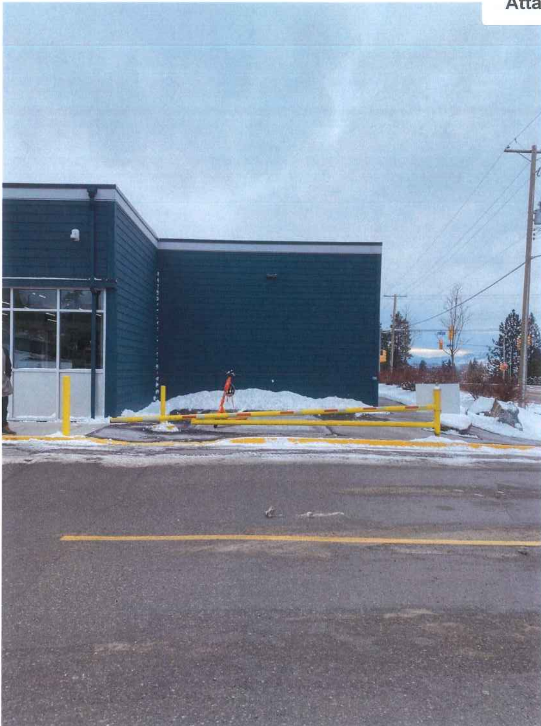
Photo 1: North Exterior – facing the parking lot
