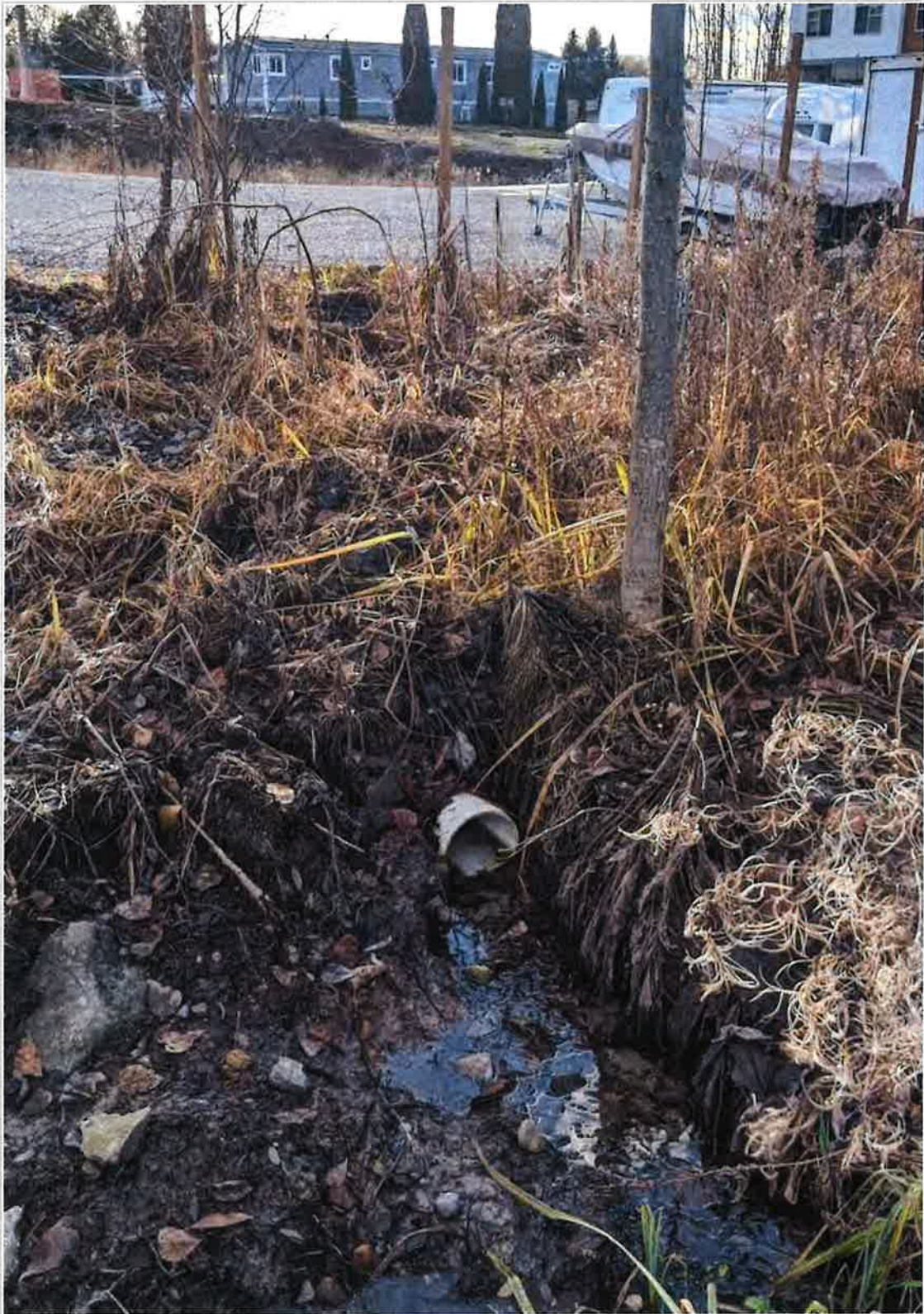
Photo 5. View of subsurface site drainage in neighbouring property (facing S ) – Nov 26, 2021.
