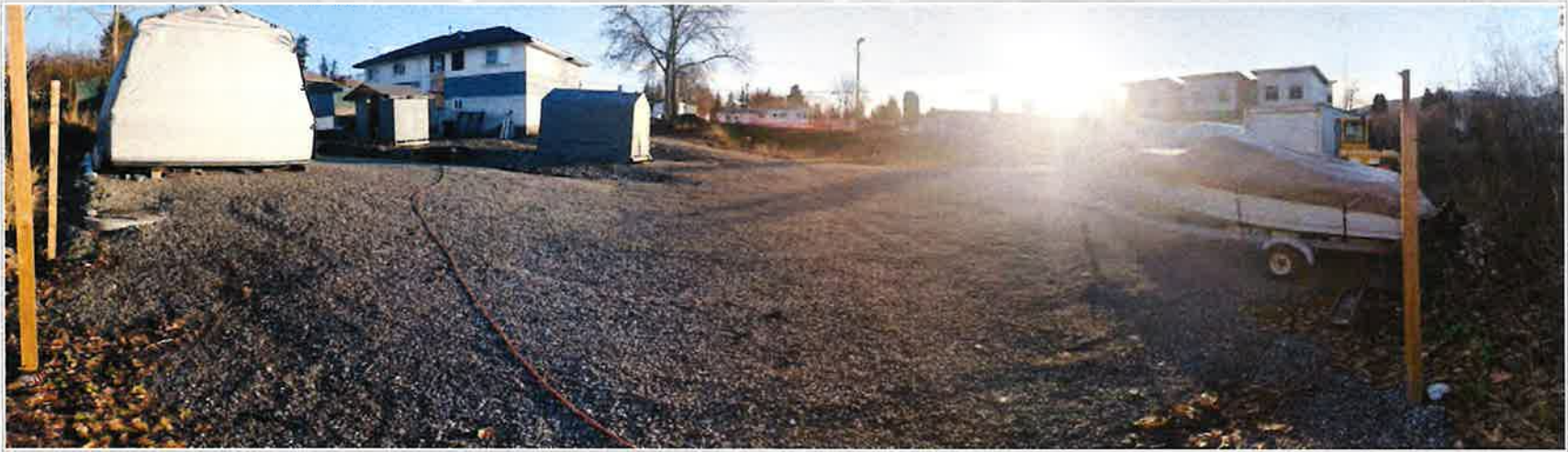
Photo 1. Wide angle view from the centre of subject property standing on the N property line (looking S) – Nov 26, 2021.
