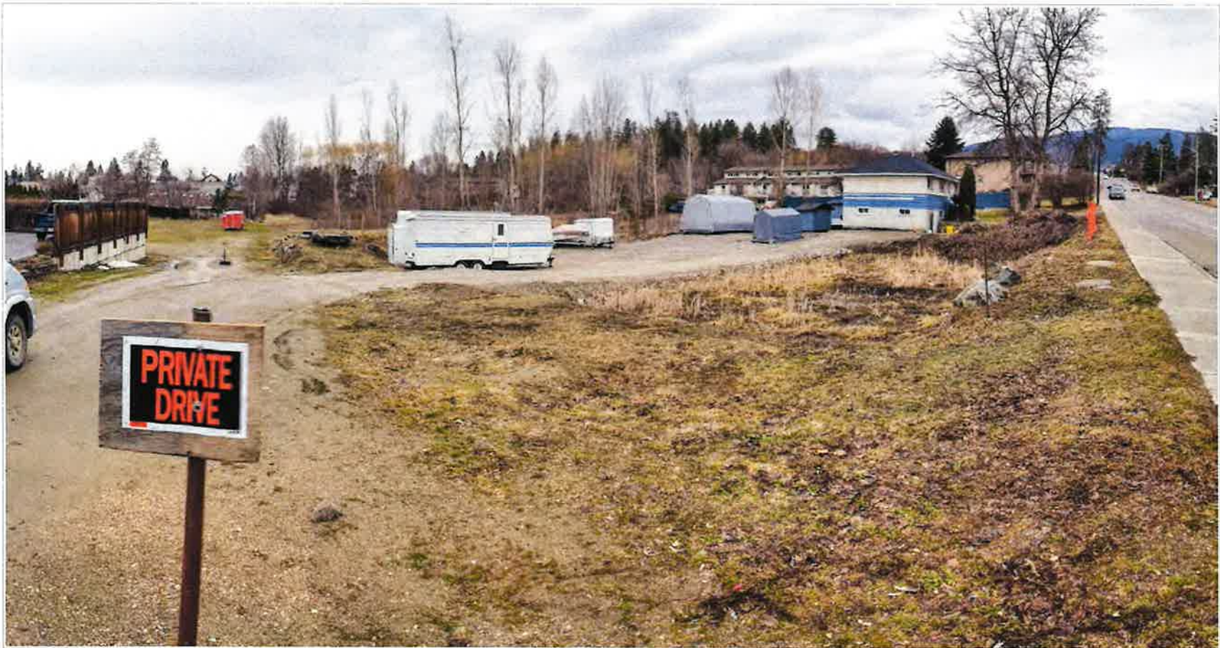
Photo 2. View of subject property from SW corner, berm containing City installed storm drain along west property boundary (small trailer parked on north end) and limiting water movement through the subject property, damp depression with cattails located right of centre and chestnut tree beyond (looking NE) – Mar 17, 2022.
