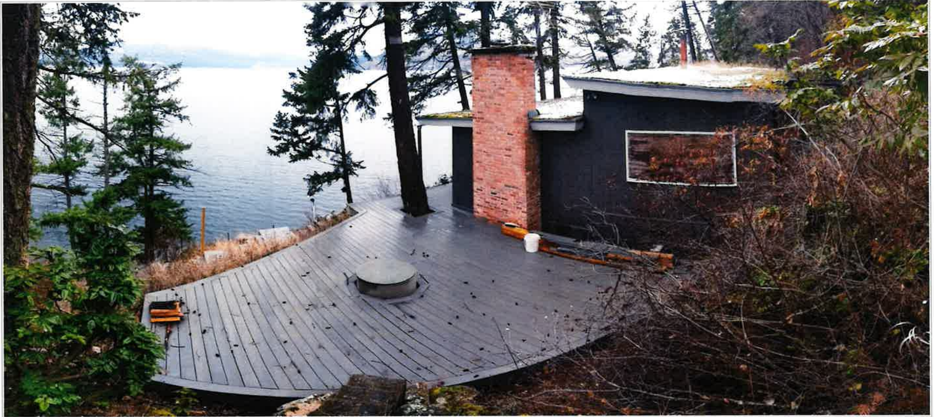
Photo 4. Existing deck and residence (from concrete steps - looking N) – Dec. 14, 2020.
