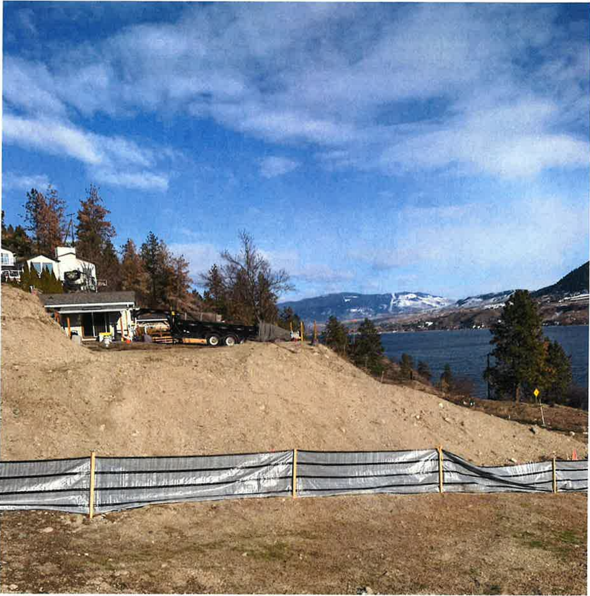
Photo 2: Site fill and grading
