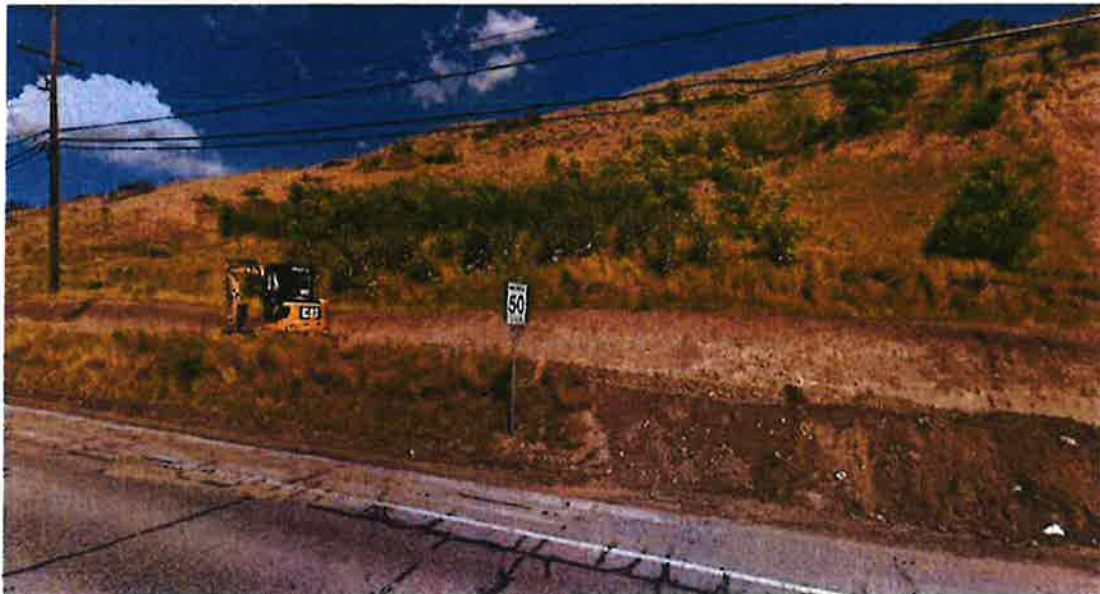
Figure 2: Street view of approx. proposed building locations, from Kalamalka Lake Road
