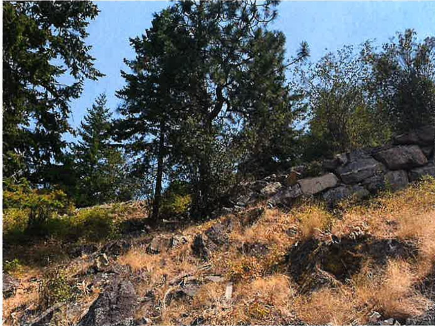
Photograph 7. View upslope the built rock wall and rock outcrops on the lower portion of the Property outside of the development footprint (July 20, 2021).
