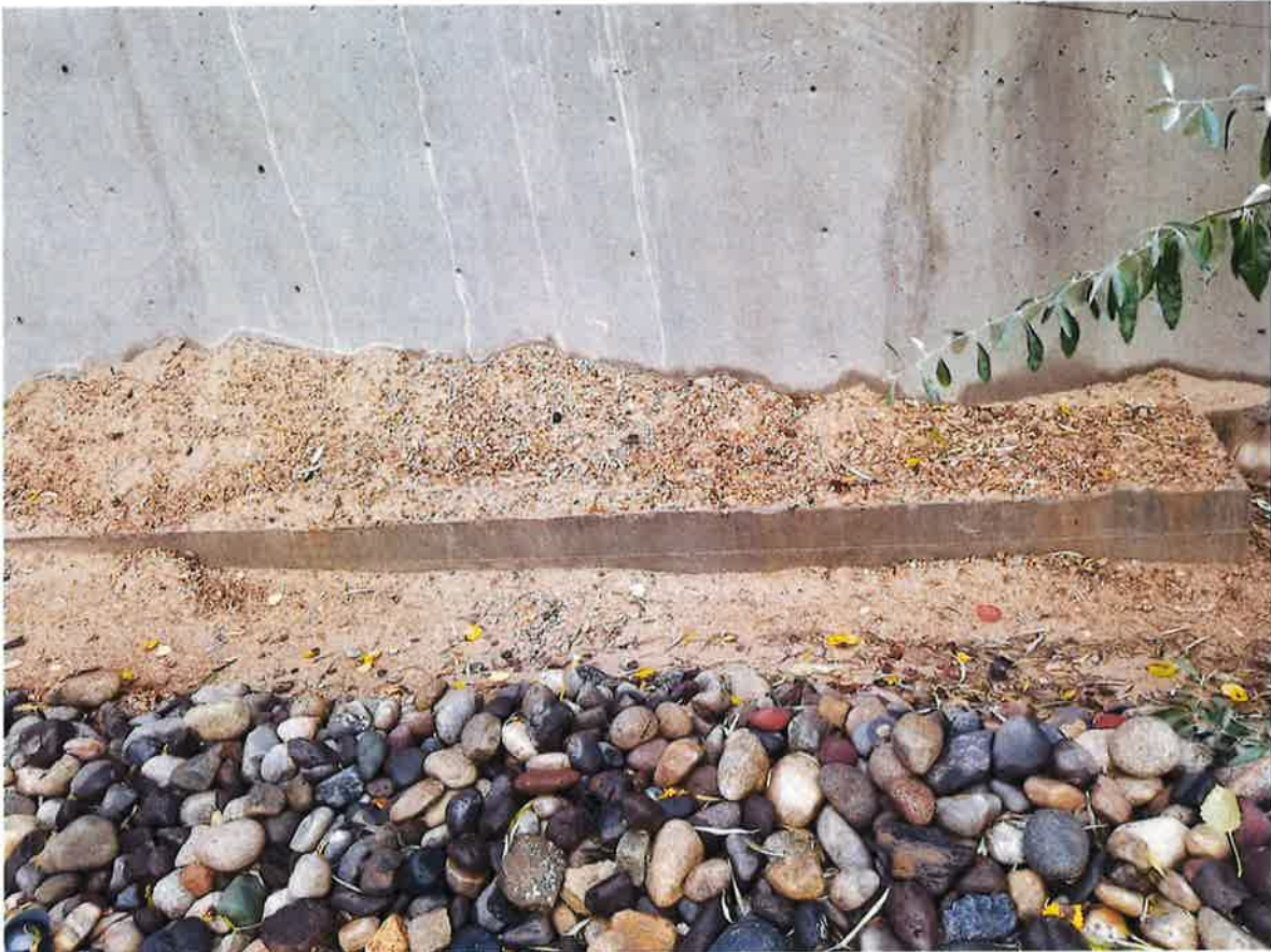
**Shows the footings exposed
