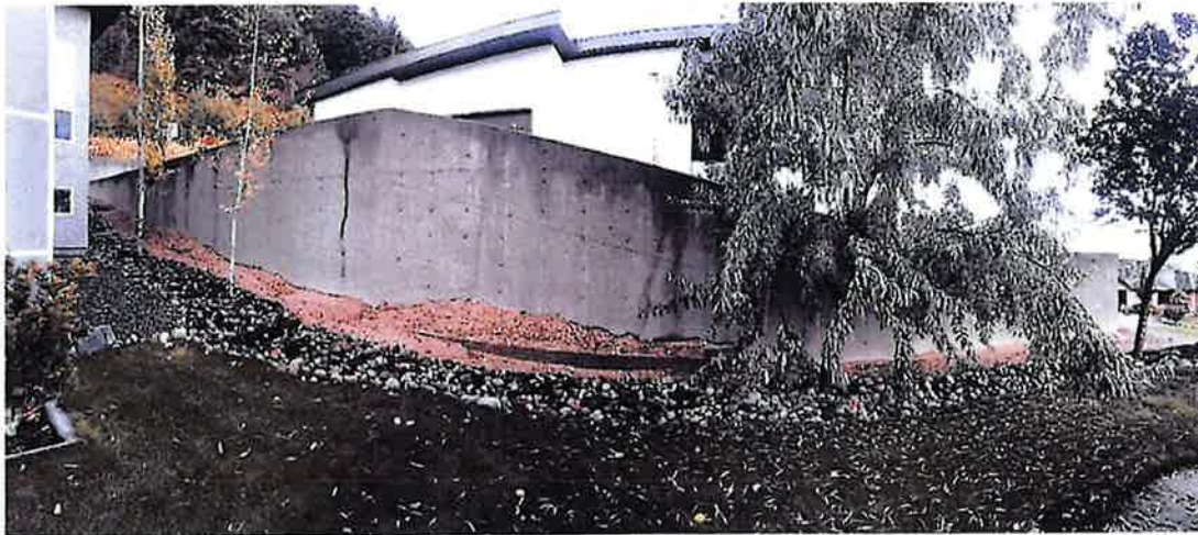
Figure 2: WE site photo of the retaining wall
