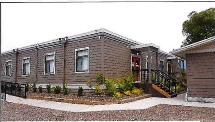
Figure 5: “Our Place” Temporary Shelter at 2307 43 rd Street
