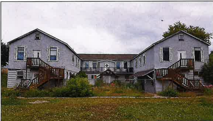
Figure 3: Front of Howard House at 2307 43 rd Street (to be demolished)
