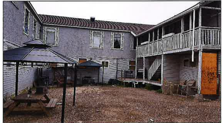
Figure 4: Back of Howard House at 2307 43 rd Street (to be demolished)
