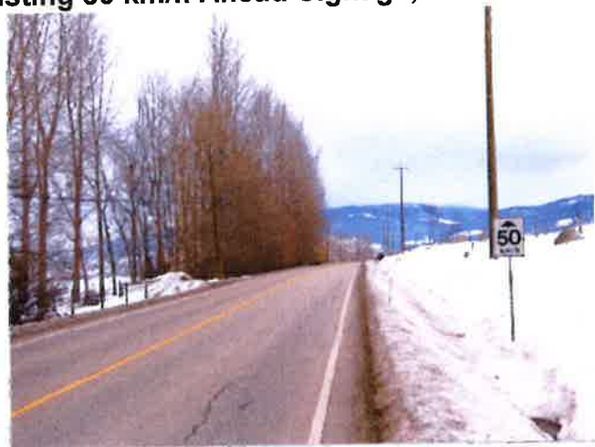
Figure 4: Existing 50 km/h Ahead Signage, Mission Road Northbound
