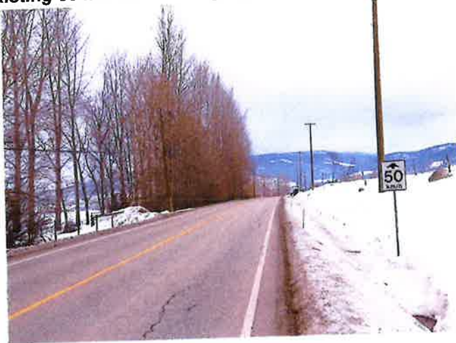
Figure 4: Existing 50 km/h Ahead Signage, Mission Road Northbound
