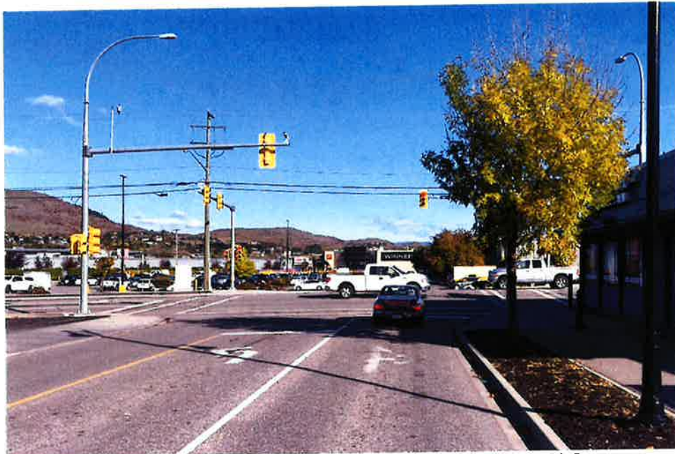
Figure 22: Issues with Primary Signal Head Visibility – 48 Ave at 29 St
