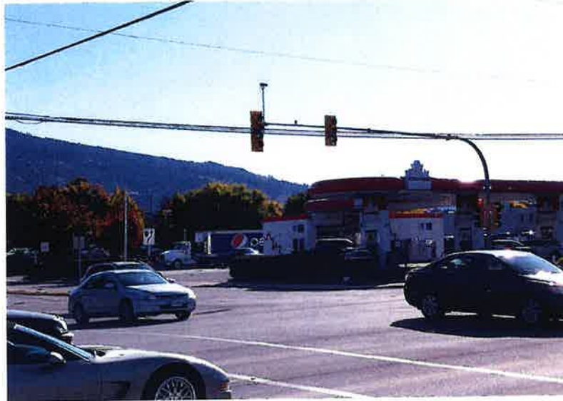
Figure 4: Powerlines Through Signal Displays – 48 th Ave at 27 St
