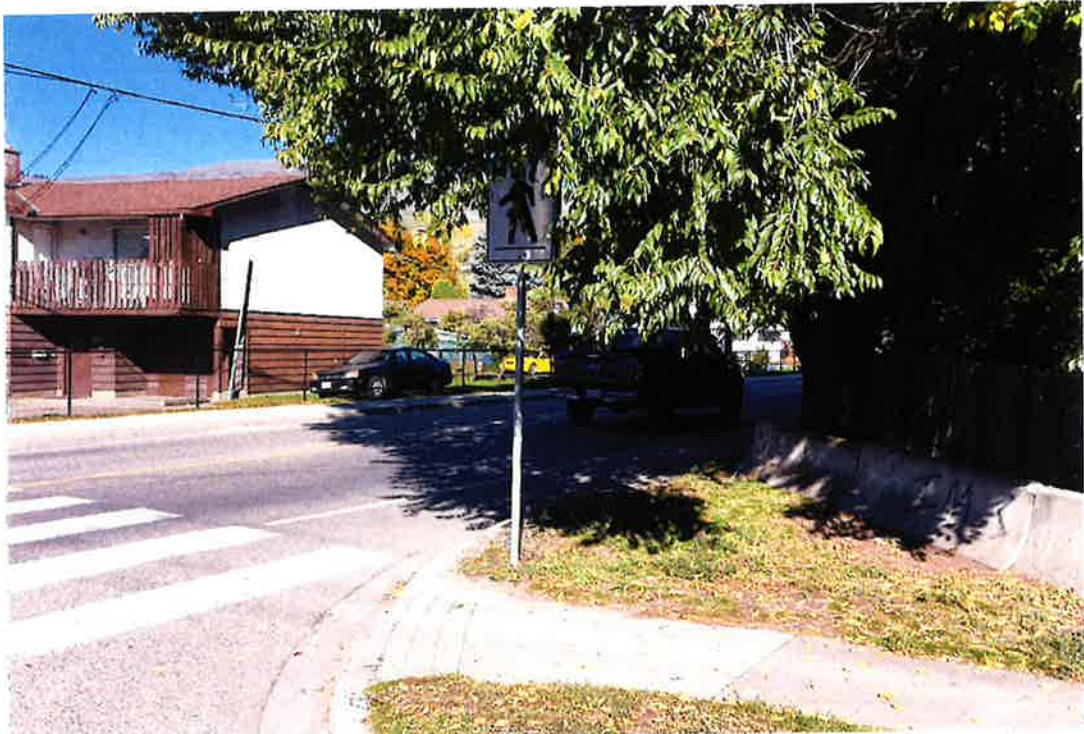
Figure 24: Obstructed Sight Lines and Signage – 27 Ave at 41 St
