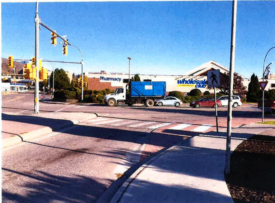
Figure 14: Existing “Smart” Channelized Right Turn – 43 Ave at 20 St
