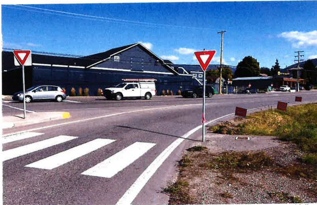
Figure 16: Yield Signs at Short Merge Lane – 48 Ave/Silver Star Rd at Pleasant Valley Rd
