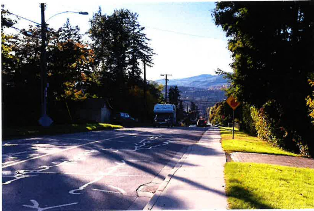
Figure 38: Obscured Westbound Stop Ahead Sign – 39 Ave at Pleasant Valley Road
