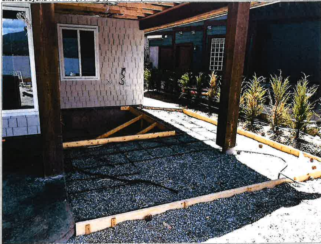
Photo 8. Concrete beneath roof removed to create sunken hot tub location. New concrete will NOT extend beyond roof line (looking S) – June 11, 2019.
