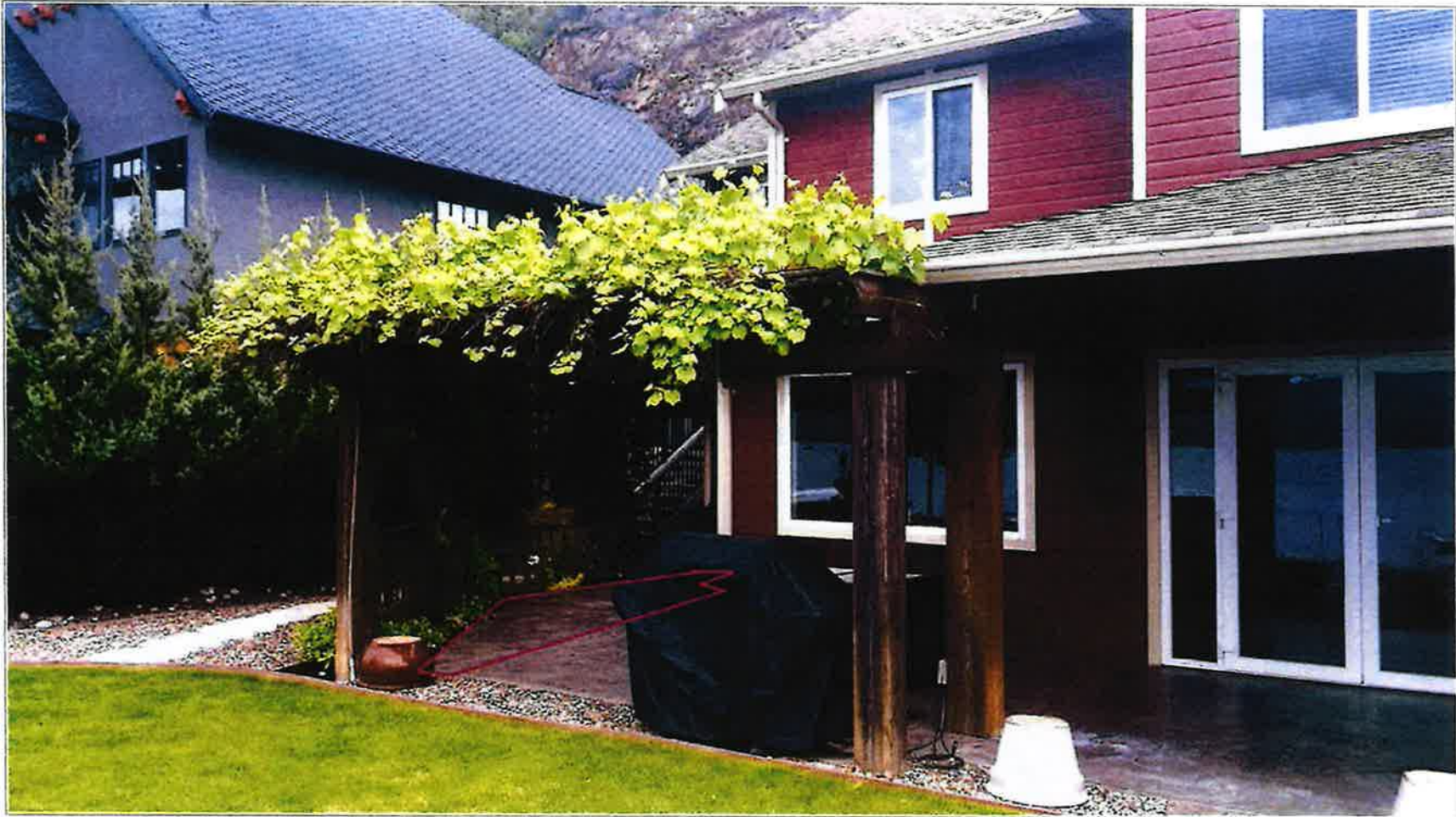
Photo 5. View of portion of existing uncovered deck that have been removed, in magenta (looking SE) – May 18, 2018.
