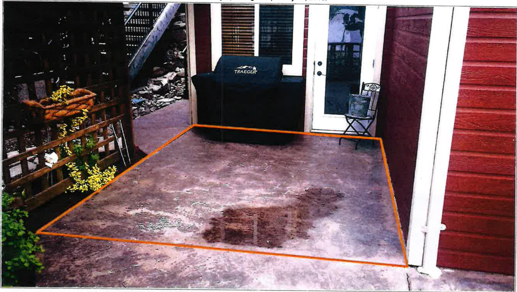
Photo 4. View of the initially proposed kitchen addition area in orange (looking SSE) – May 18, 2018.
