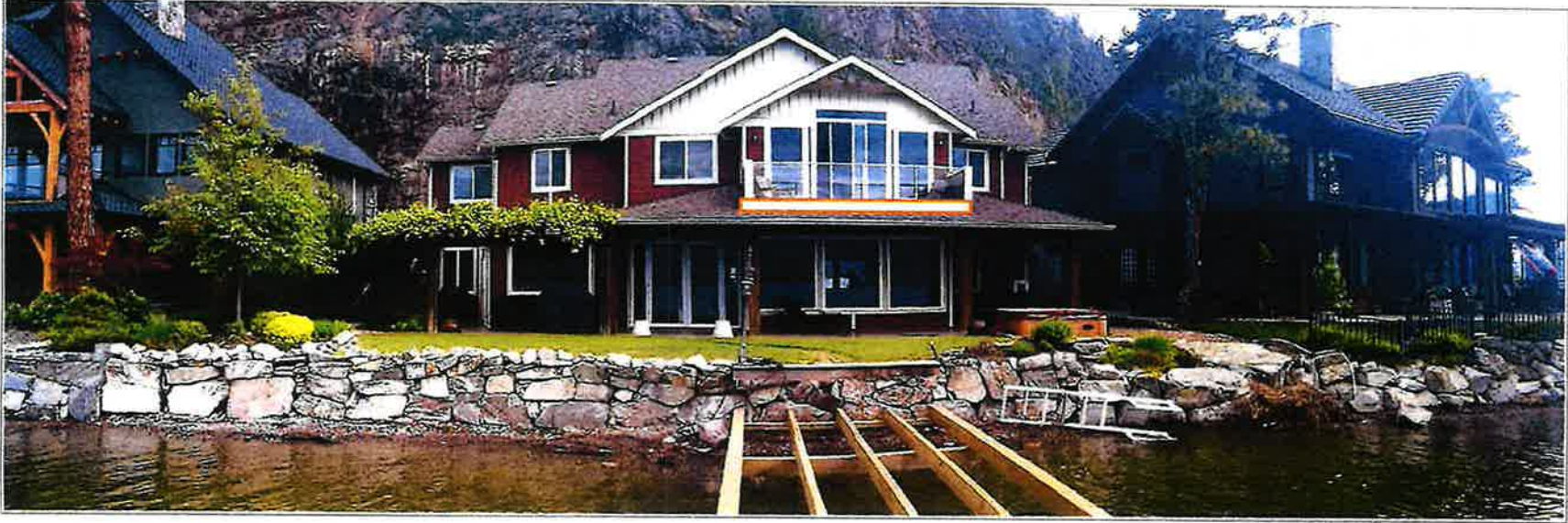
Photo 1. View of the Subject Property, and foreshore from near the end of the existing dock, with the proposed enclosed second floor deck area (looking SSE) – May 18, 2018.
