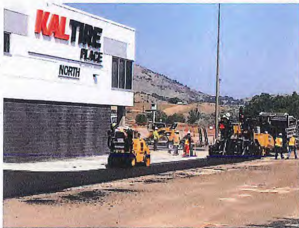
Paving – Crew works to pave the east side of the new building.
