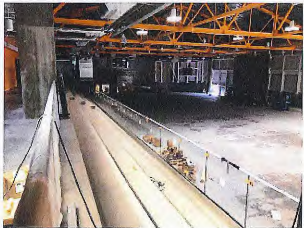
Bleacher Glass – new higher glass is installed in the bleacher area.
