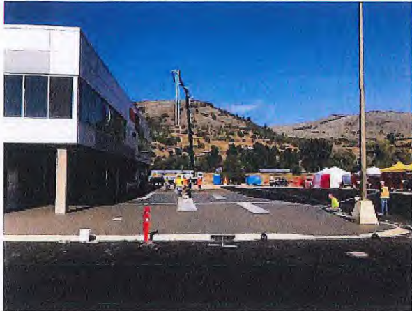
Plaza – Concrete for the plaza in front of the new building has been poured..
