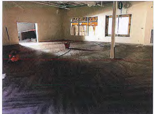
New Flooring – Flooring is installed in the new Civic Room which is part of the transition area.
