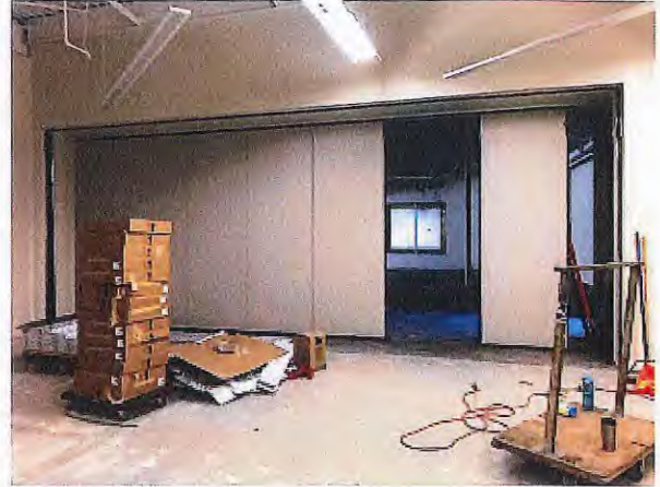
Movable Wall – The movable partition wall has been installed in the transition area.
