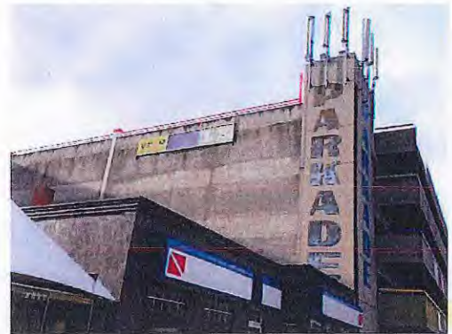
Existing signage – north side.
