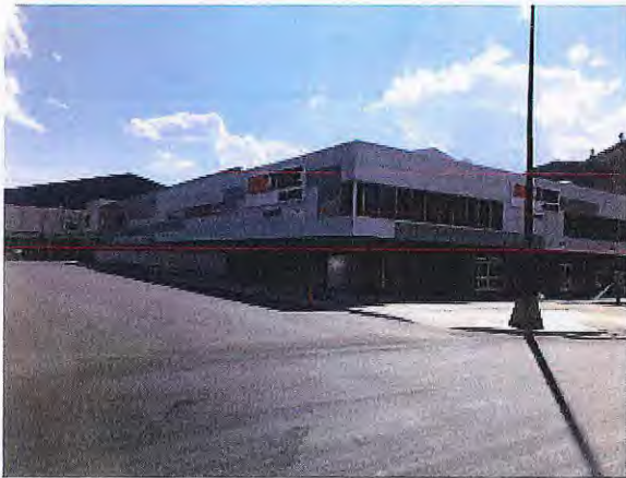
Paving – Paving has been completed on both the east and north sides of the building.
