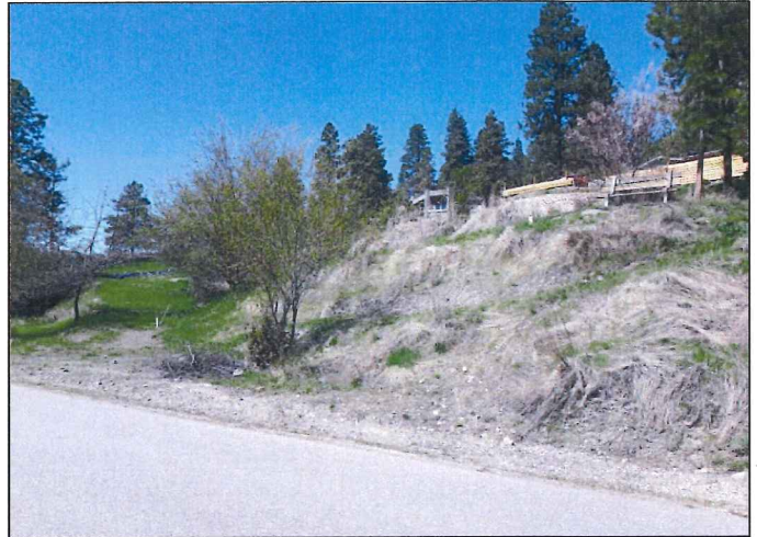
Figure 4 – Nature of Existing Slope on Property
