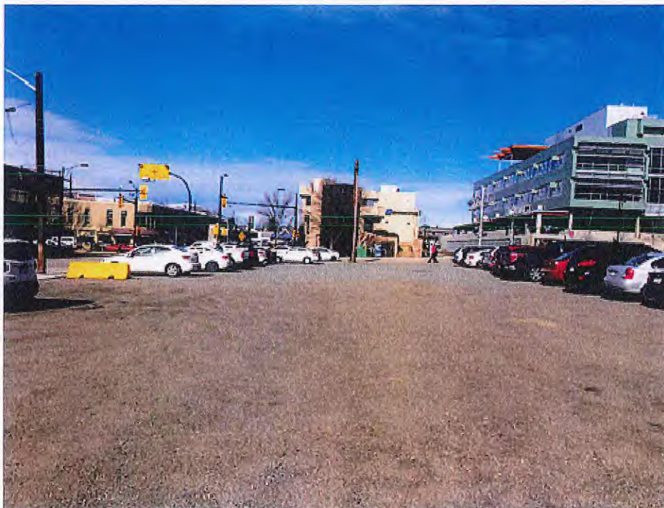
North half of parking lot surfaced in recycled asphalt pavement (RAP)
