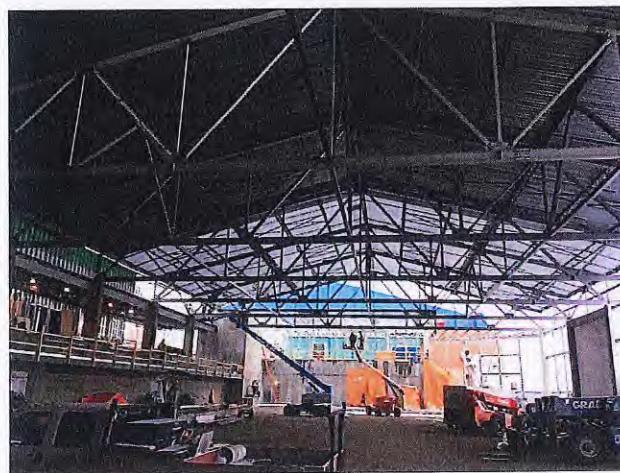
Arena Roof – Q decking now fully installed on main arena roof and sprinkler system being installed.
