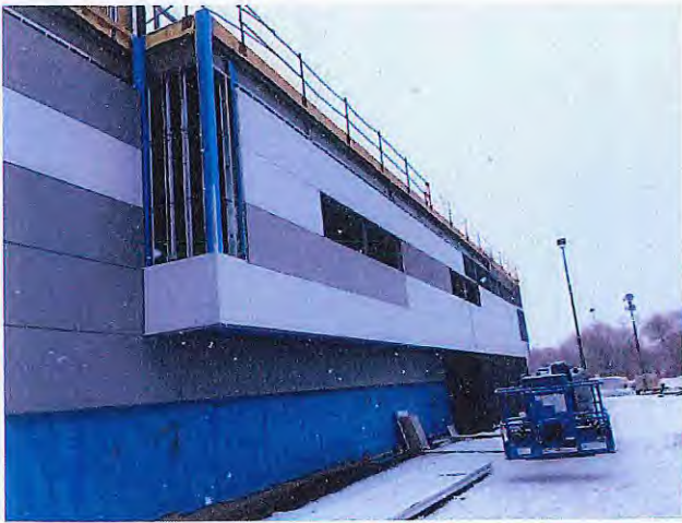
Kingspan Siding – Kingspan Siding is installed on the east side of the facility.
