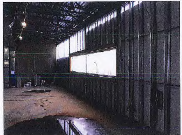
Kingspan Panels – Kingspan panels now installed on exterior provide some closure on the interior.
