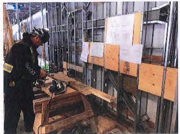
Backing – Backing for fixtures, dispensers and equipment being installed in all spaces.
