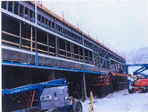
Siding Framing – the frames are being put in place for the Kingspan siding on the north end.
