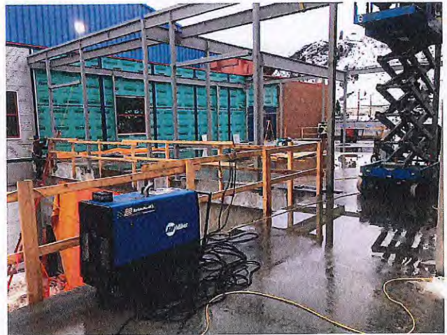
Transition Area – The transition area between the two buildings is now framed and being roofed.
