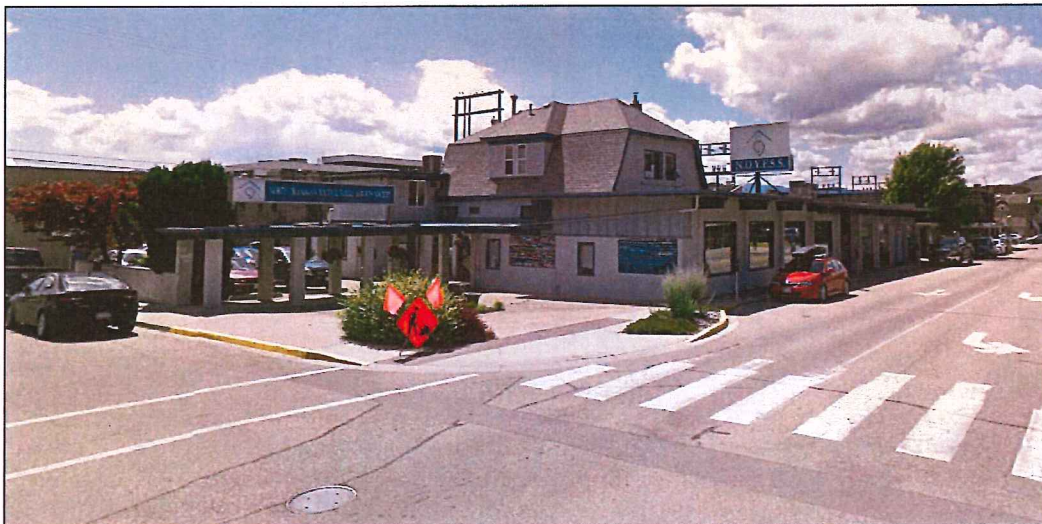
Figure 2 – Existing Building at 3100 – 32 nd Avenue
