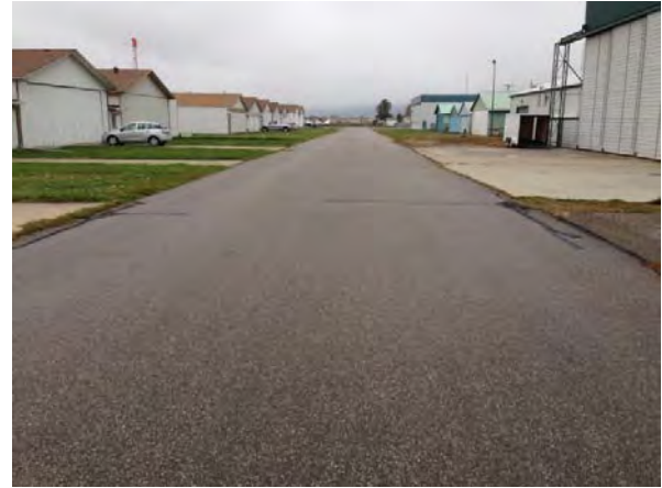
Photo 4:22 - Section 9 overview – cont'd
