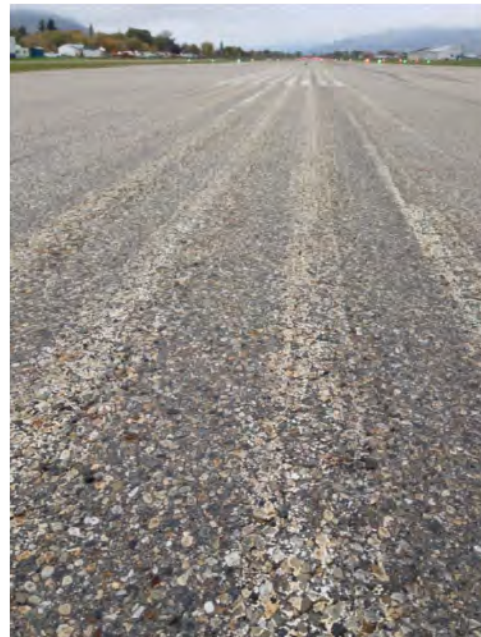
Photo 4:2 - Minor raveling in Section 1
