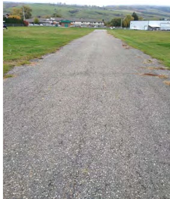
Photo 4:27 - Section 11 overview – cont'd
