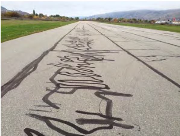
Photo 4:7 - Extensive crack sealing
