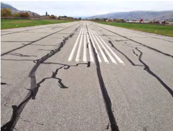
Photo 4:5 - Section 5 overview from Twy-D
