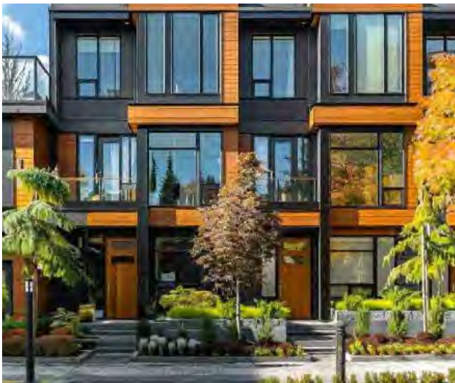
Figure 41: Design primary unit entrances to provide, a comfortable entry zone, a visible front door, and a clear transition from public to private space.
