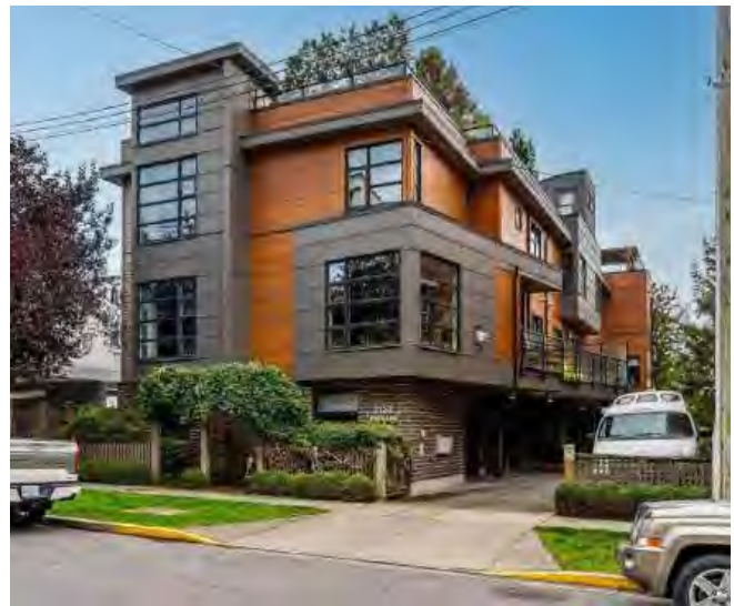
Figure 42: For buildings oriented perpendicularly to the street, establish a strong street relationship with the end unit.
