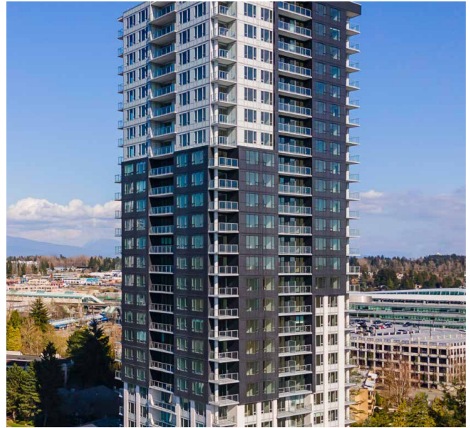
Figure 50: Example of tower middle.
