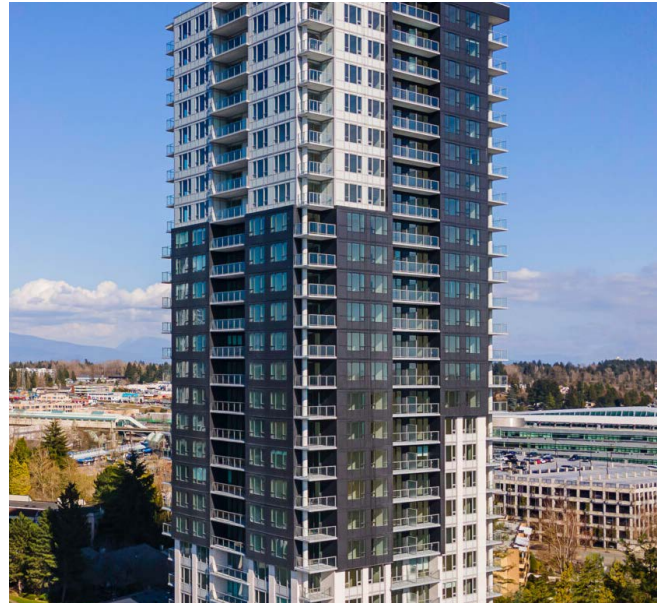
Figure 50: Example of tower middle.
