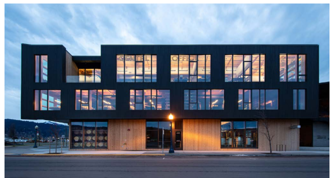
Figure 55: Use different exterior materials to distinguish the warehouse or plant area from the office or sales area.
