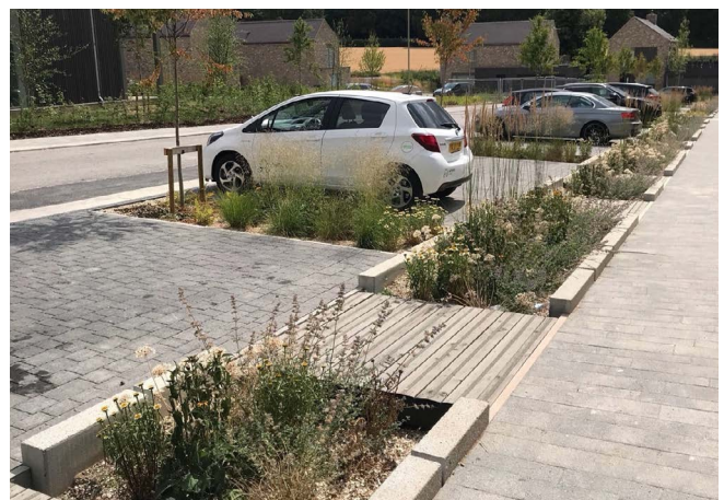
Figure 30: Design parking areas to maximize rainwater infiltration.
