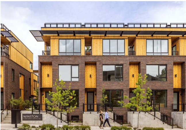
Figure 11: Incorporate high quality, natural materials like wood, stone, and masonry into building facades, while maintaining FireSmart principles.
