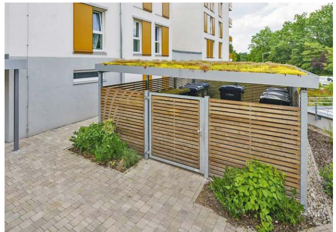
Figure 16: Locate 'back-of-house' functions (such as loading areas, garbage collection, utilities, and parking access) away from public view and separate from pedestrian circulation routes.
