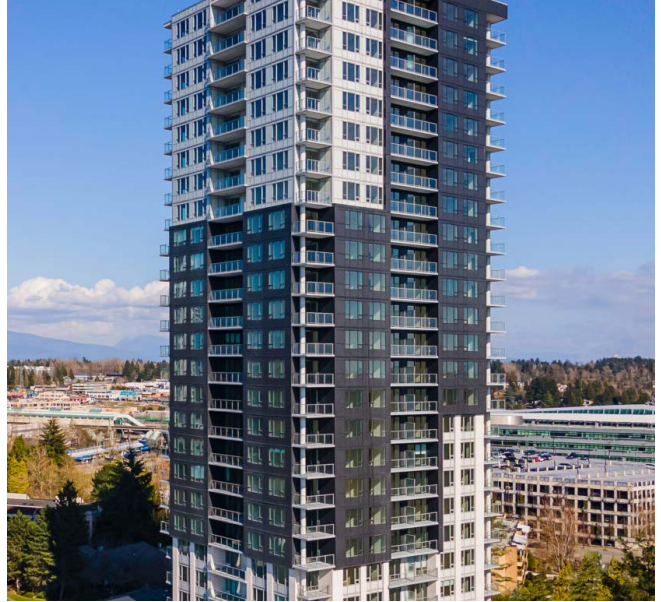
Figure 50: Example of tower middle.
