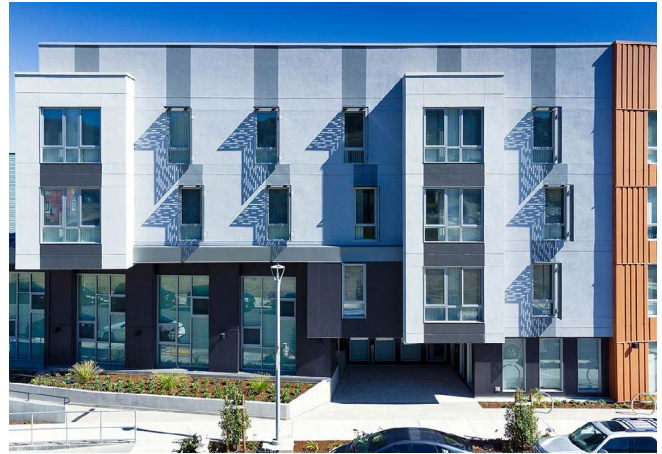
Figure 35: Use exterior shading devices to block excess heat gains in summer and allow passive heat gains in winter.
