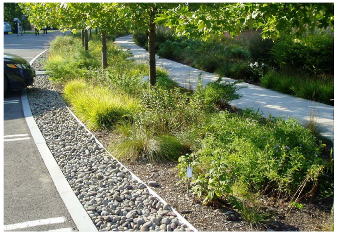
Figure 53: Provide on-site bio-retention facilities (e.g. bioswales, rain gardens) to collect, store, and filter stormwater from parking areas.
