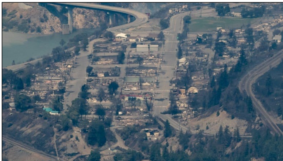
Figure 19. Image of Lytton, BC, after the 2021 wildfire showing unburned vegetation surrounding destroyed homes and structures. Source: CBC.
