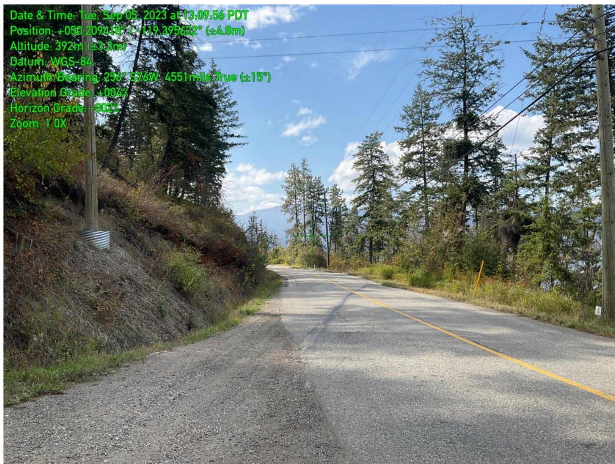
Figure 4. Example of wooden power poles located on an egress route within the CWRP AOI.
