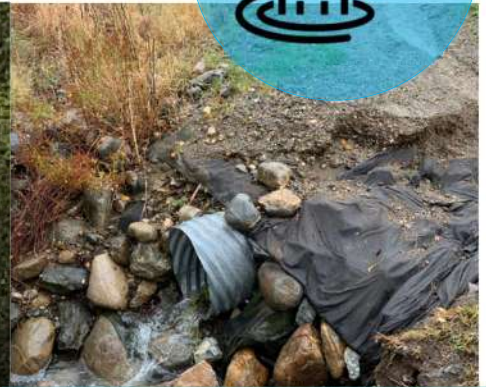
Washed out culvert/pathway - Foothills
