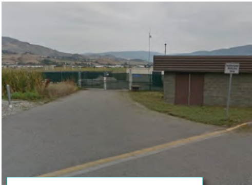
Cummins Road Pump Station
