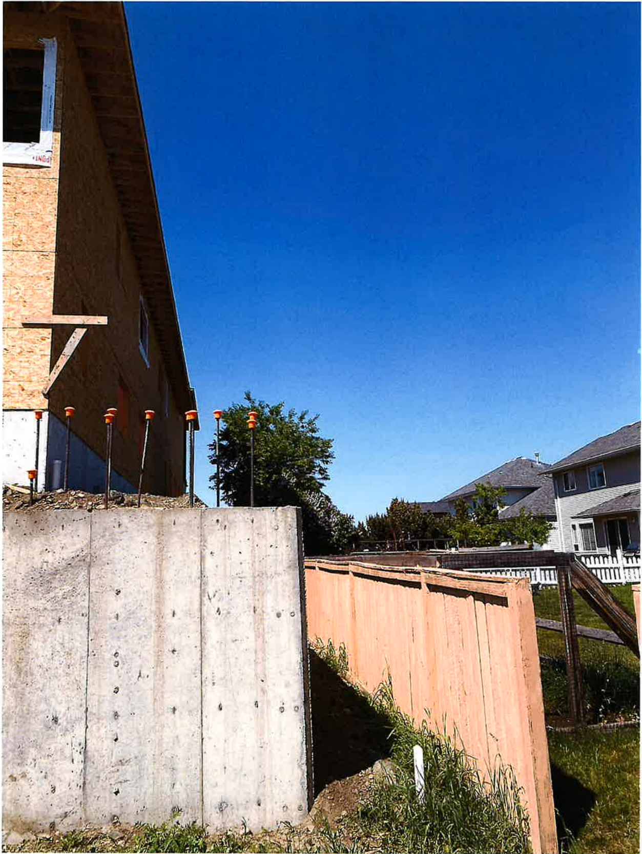
Photo 2: Existing retaining wall height rear SE corner
