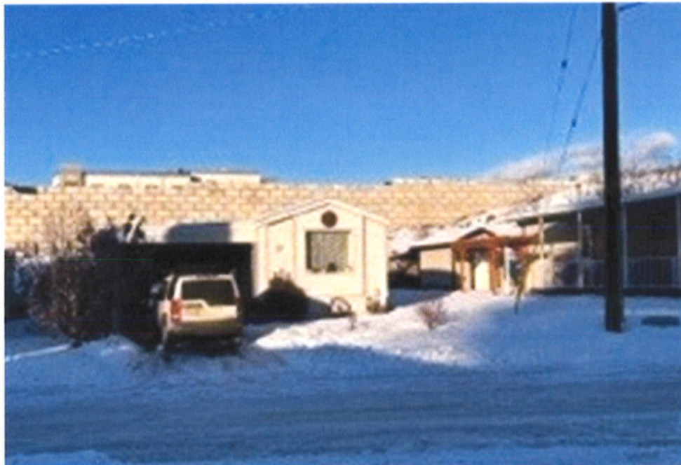
Silver Star Gateway Lock Block Wall Along North Property Line
