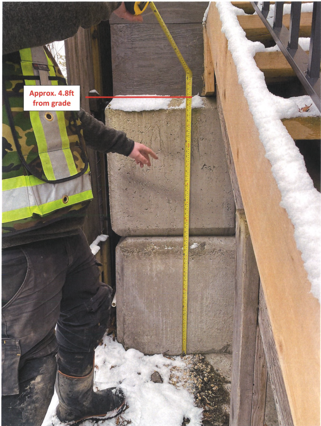
Photo 7: Retaining wall height at rear (NE corner) between 7373 & 7349 Brooks Lane
