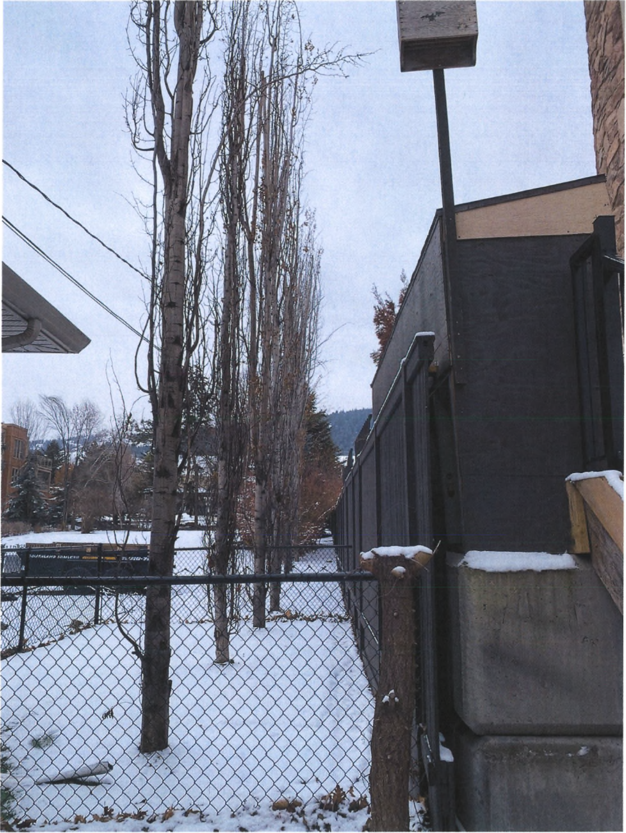
Photo 6: Existing retaining wall/fencing at rear (NE corner) between 7373 & 7349 Brooks Lane
