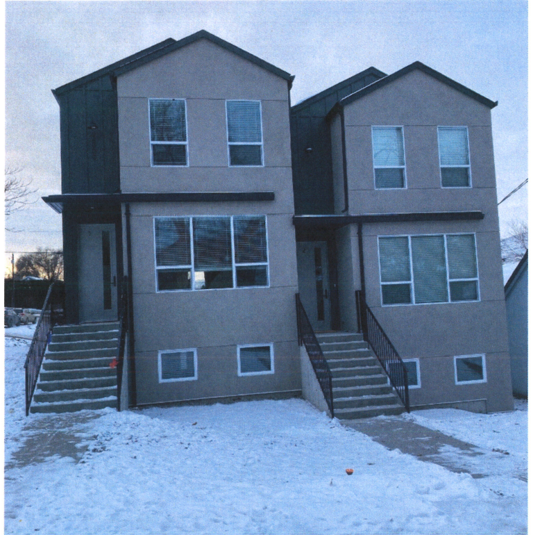
Photo 1: 2000 33 rd St (2021/semi-detached/unit width variance from 7.5m to 5.5m)
