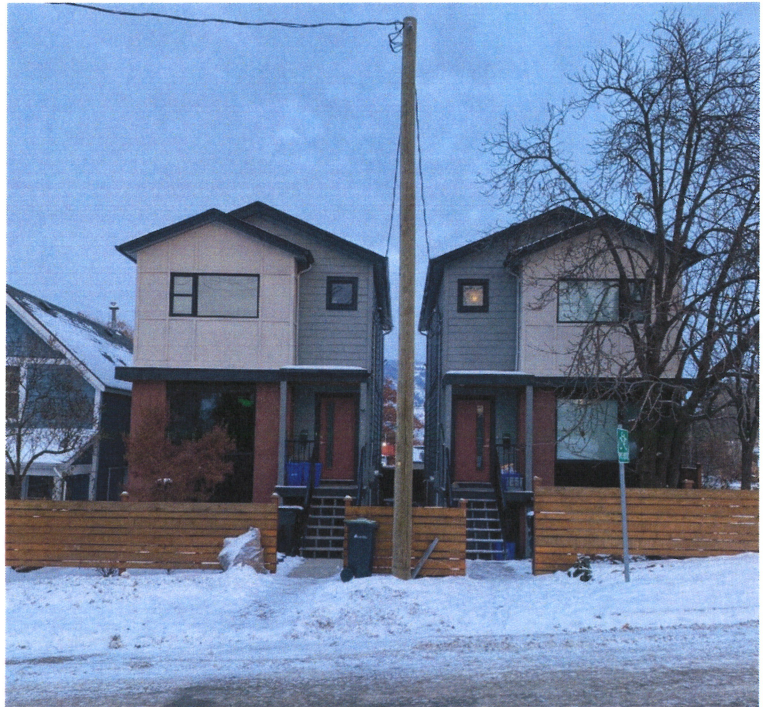
Photo 3: 1601 33 rd St (2017/2 SDH & suites/unit width variance from 7m to 5.4m)
