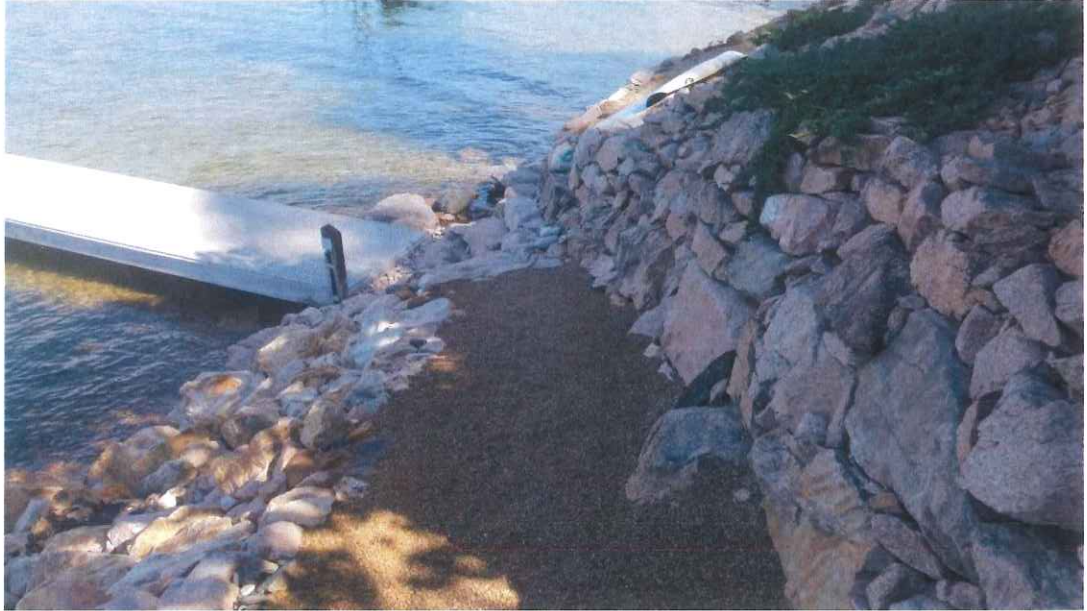
P1 Photograph 1. Existing pathway (July 22, 2020)
