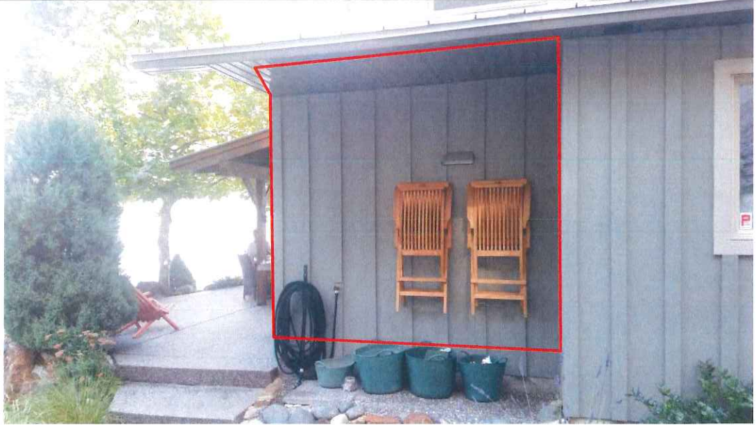
P2 Photograph 2. Approximate cantilevered kitchen addition location (red outline) (July 22, 2020)
